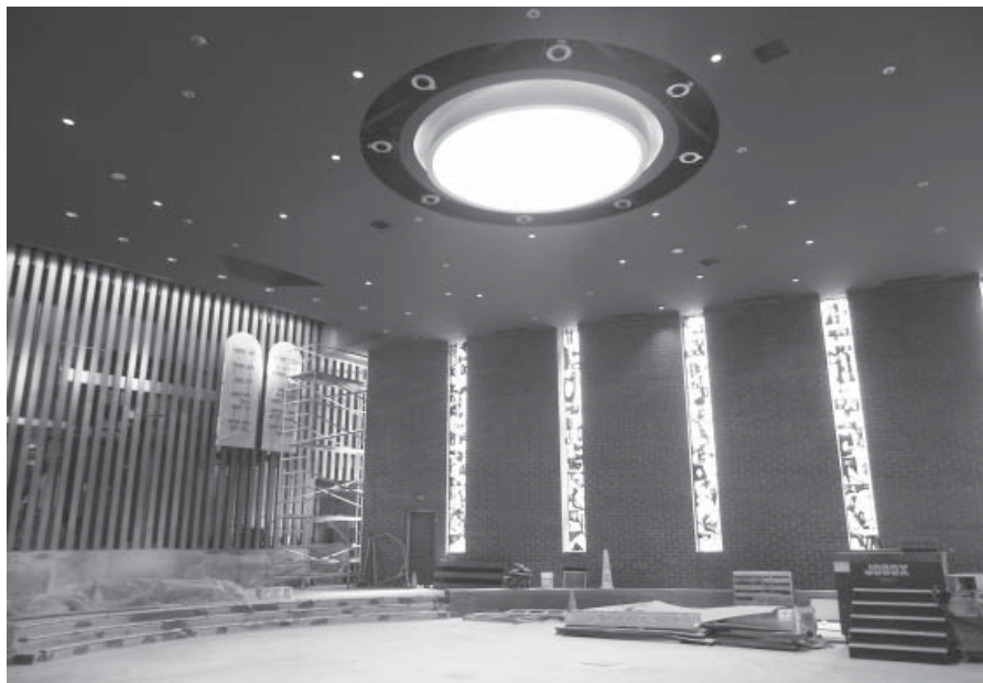
Sanctuary under construction
